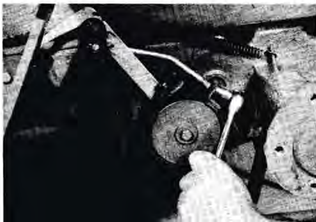
FIG. 8 — BRAKE ADJUSTMENT
