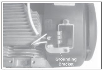
Figure 11-71. Grounding Bracket and Attached Connector.
